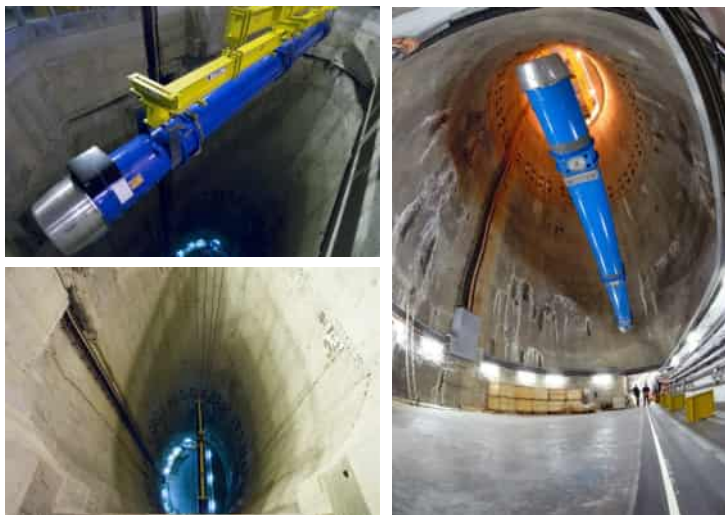
Figure 1.12: The challenge of lowering 1232 dipole magnets to the LHC tunnel. Each dipole weighs 34 tonnes and is 15m-long. Technicians and engineers worked days and nights, carefully installing 20 magnets a week between March 2005 and April 2006. Once they have been lowered down through a single specially constructed shaft, they begin a slow progression to their final destinations in the LHC tunnel, taking about 10 hours to arrive at the furthest point on the LHC ring.
