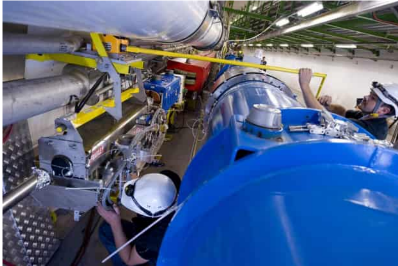
Figure 1.18: Installation of a collimator in a LHC injection line (23 June 2009).
